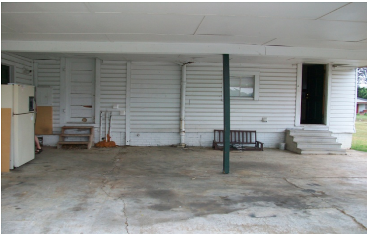
Figure 5. Car port- pressure washing and fill cracks
