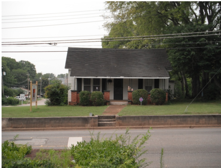
Figure 1. The Studio 1001 Oakwood Ave
