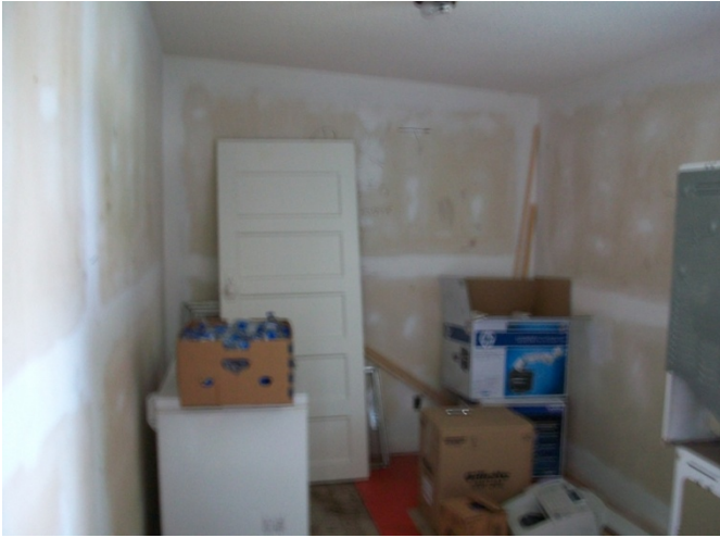
Figure 4. Locker room- paint and install shelves
